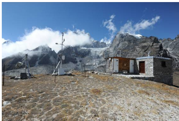
Figure 1. The NCO-P GAW-WMO Global Station after the upgrade.
